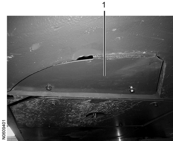
Figure 5 Inspection cover, underside of counterweight
