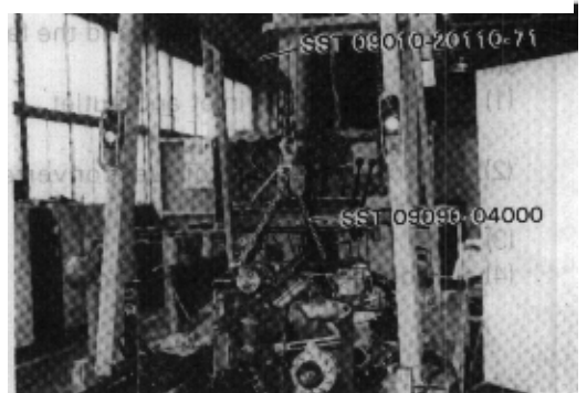
Fig. 1-20 Slightly lifting the engine
